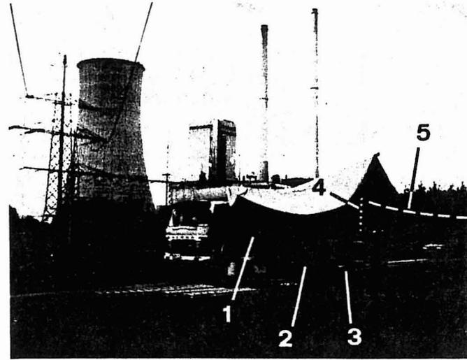
Fig. 4 . Two-Stage Testing on Site Schwandorf, Bayernwerk AG, Munich (FRG), with Live HV-Parts Unloaded and Ready for Test under Rain Sheltering Tent:
