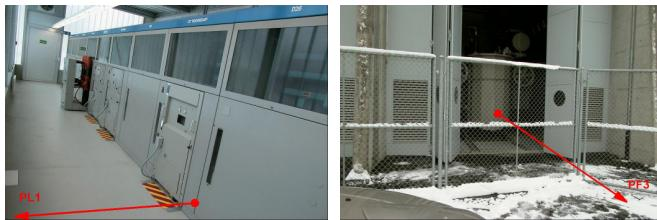
Figure 7. MV switchgear (left) and transformer (right), measuring profiles
